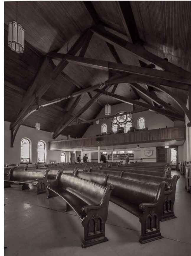
Left: before photo inside the church showing the original roof structure
