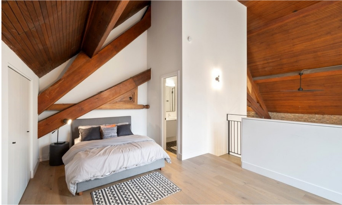
Above: loft space showing the exposed roof structure.
